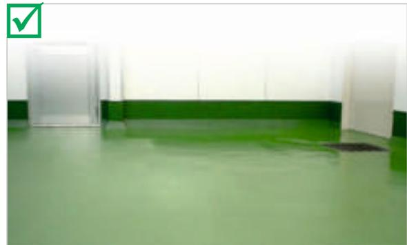
Floor with drainage of appropriate slope
