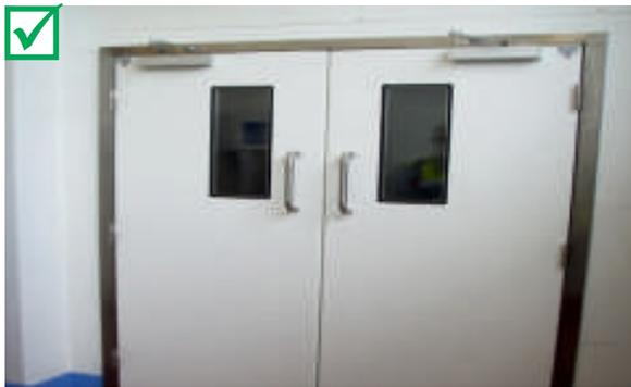
Doors made of smooth and non-absorbent surfaces
