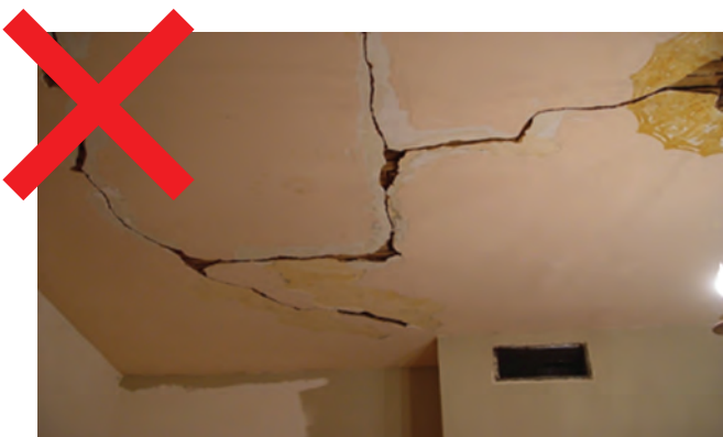
Fig. 2.25 Cracked Ceiling
