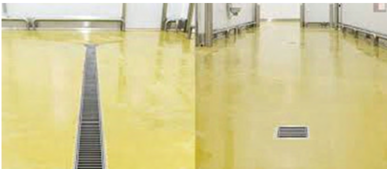
Fig. 2.10. Floors to be sloped to ensure easy drainage
