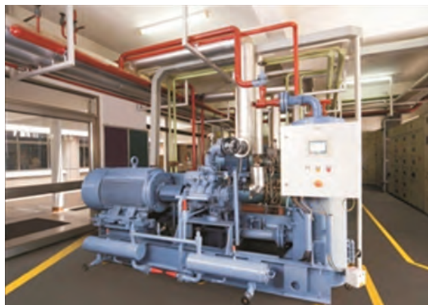
Fig. 2.30 Standard colour code for utility lines
