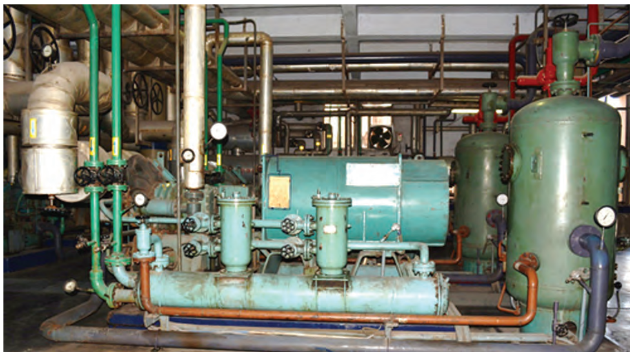
Fig. 2.31 Screw Compressor Refrigeration Plant
