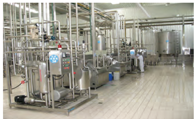
Fig. 2.24 Tiled floor to resist chemical action
