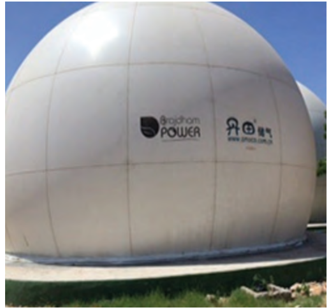
Fig. 2.36 Double Membrane Balloon for Purified Biogas
