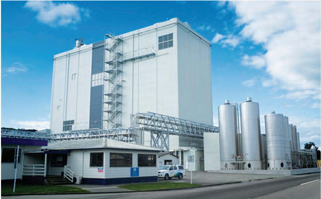
Fig. 2.18 Premises with tar road and RCC hard park to minimize entry of dirt/dust in Production area
