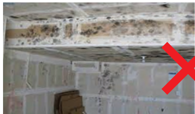
Fig. 2.26 Fungus infected Ceiling
