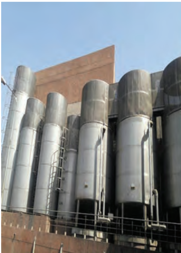
Fig 3.11 –typical bird- proofing on silos to avoid contamination
