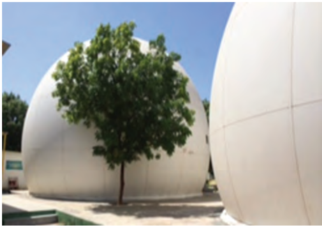
Fig. 2.36 Double Membrane Balloon for Purified Biogas
